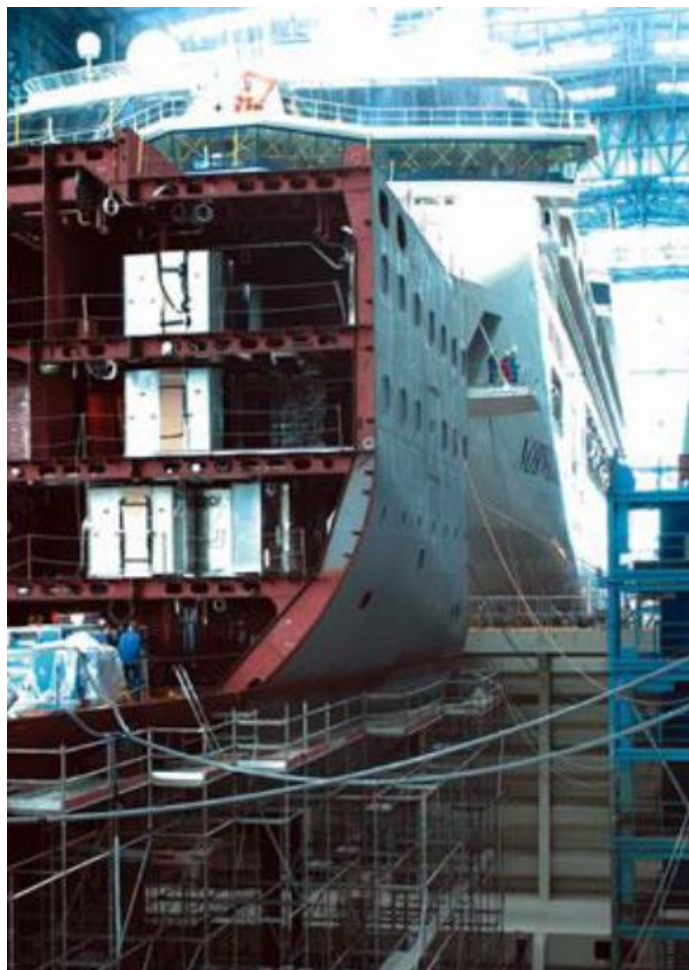
(c)激光焊接分段合拢
